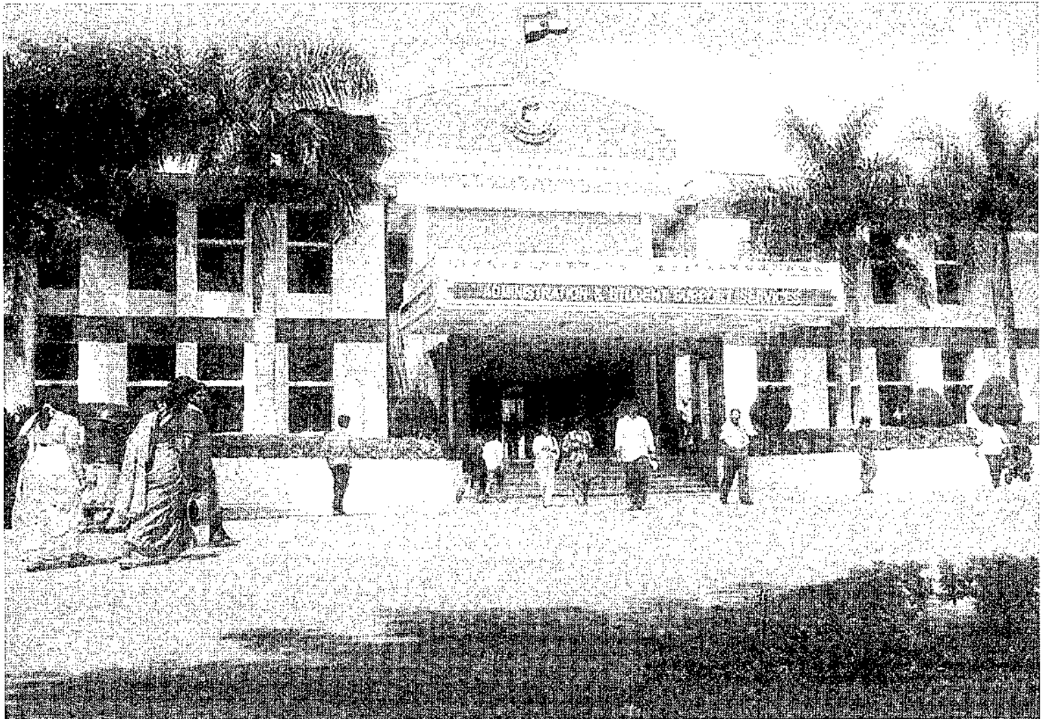
University Administrative Building
